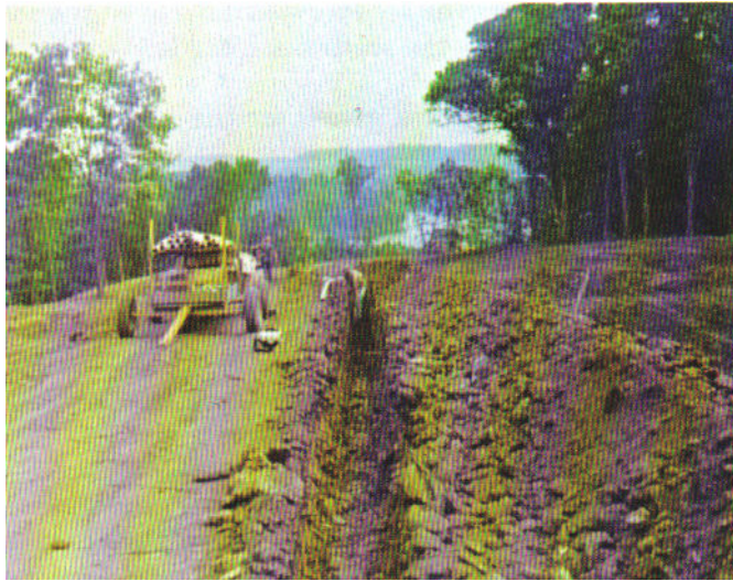
Irrigation pipe being installed on 7 th fairway.
