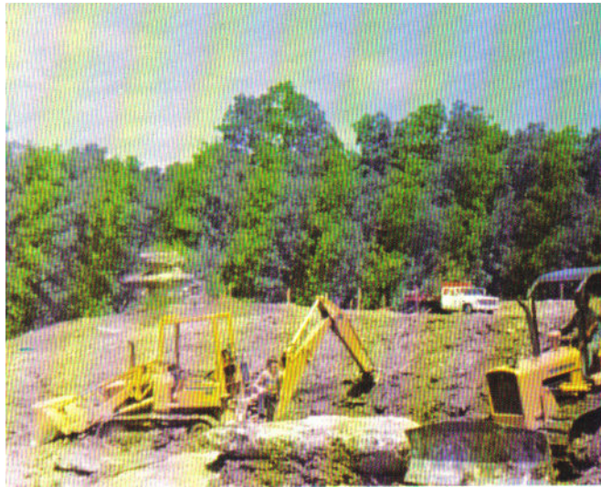
Construction of 8 th green; equipment in foreground placing rocks around the lake edge. Note: Distinctive rock outcropping now in the middle of the sand trap.
