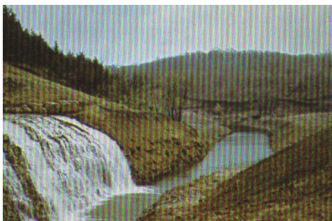
The spillway showing newly constructed channel which carries water back to the original stream.
